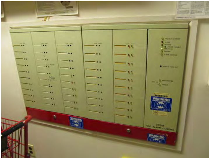
Original fire alarm control panel – Serviceable but beyond end of expected useful service life
