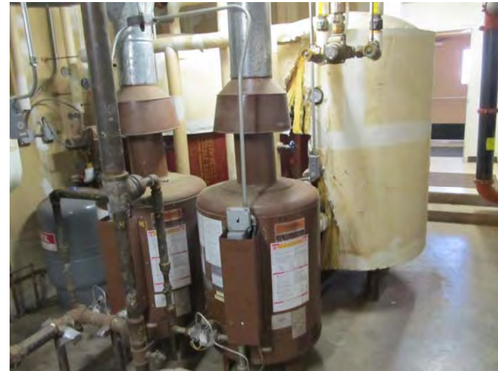
Boilers (in brown at foreground) and storage tank for building's domestic hot water system
