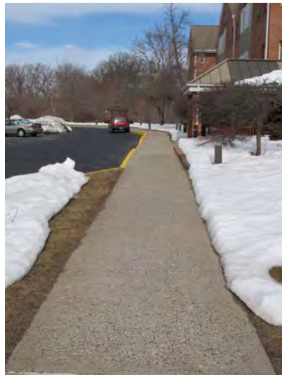
Typical concrete sidewalk – No significant damage noted
