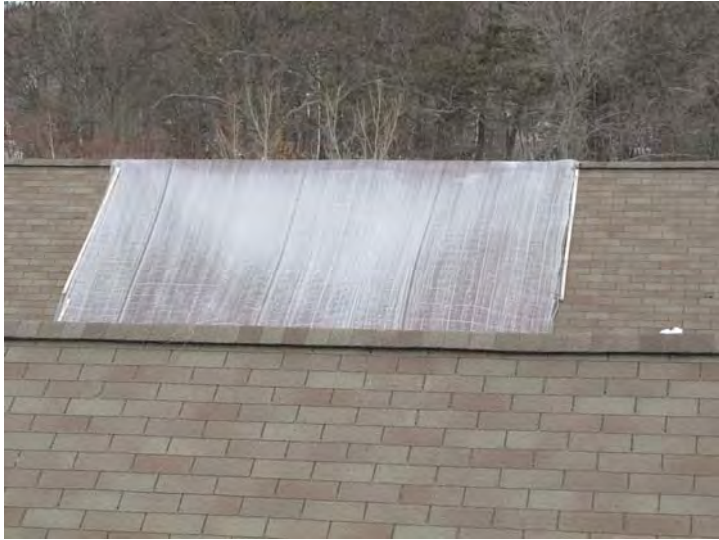
View of tarp over a section of roof where leaks have been an issue
