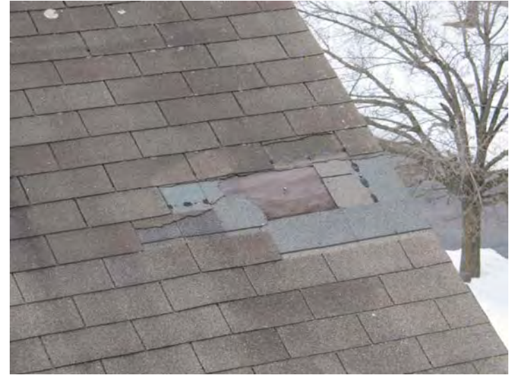
Close-up view of area where roof shingles are broken/missing
