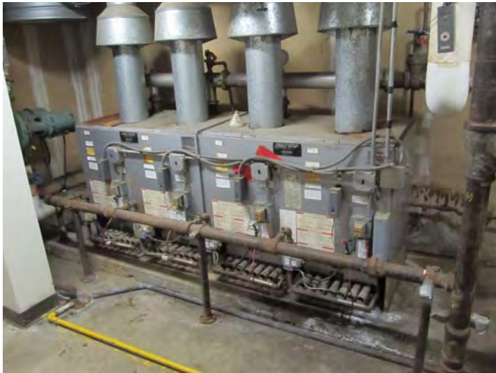
Original boiler plant for production of hydronic heat – Serviceable but nearing end of expected useful life
