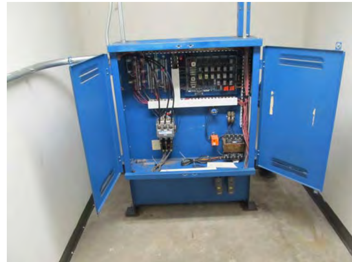
Original hydro-mechanical and controller/dispatcher equipment for building's elevator
